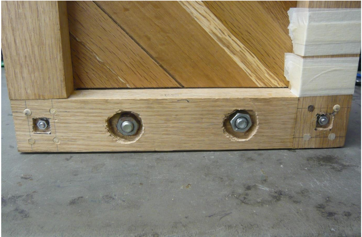
Photo 28: Close-up view of four of the counter-sunk nuts.
